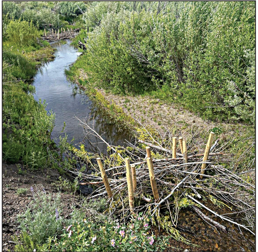
Beaver dam analog near top of project area.
